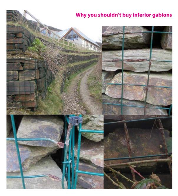
A wall constructed only a few years ago The gabions are corroding heavily beneath the pvc coated wire, we suspect very low zinc coating weights if at all. Additionally the plastic jointing clips are non conforming with industry standards.
